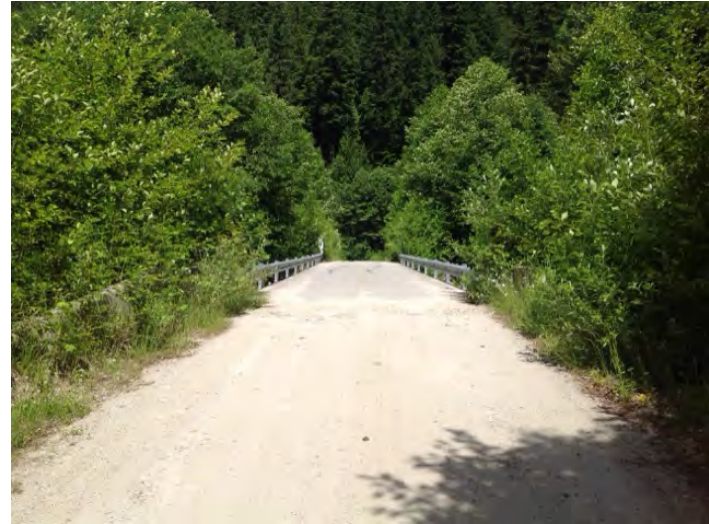
Approach from Left Bank when facing downstream
