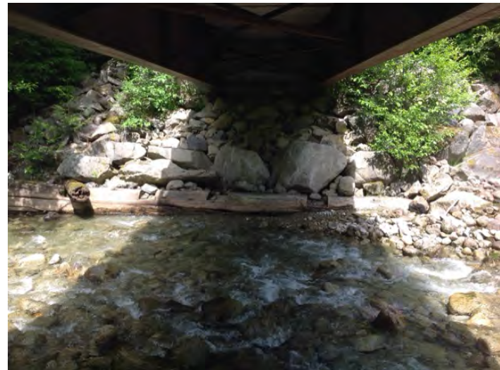
Right Bank Abutment when facing downstream
