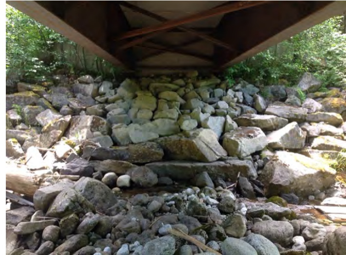
Left Bank Abutment when facing downstream
